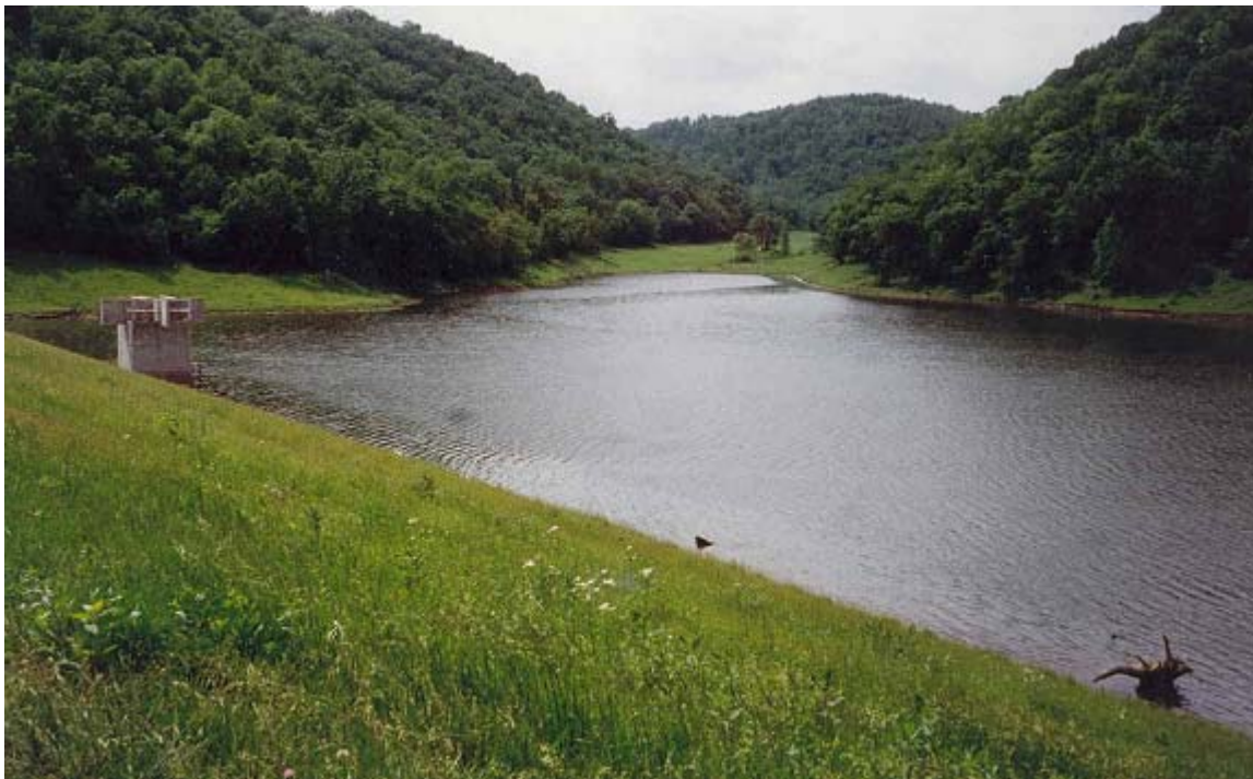
South Fork Lake in Houston County. View from dike to the Southwest, 1996.
